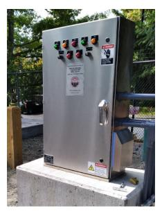
systems can be operated independently with the EEW signal providing advance warning to personnel and the MSC separately performing site specific 2/2 or 2/3 voting with a variety of sensor configurations (i.e. standard flat response, ANSI/ASCE/SEI 25 response, etc.).
