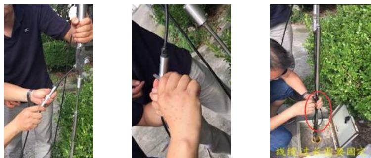
6.4 The last probe (the top one) should be connected to the steel suspension kit, and the latter be fixed to the wellhead tool on the borehole opening.
